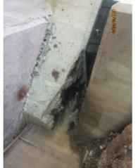
BEAM 5 AT END BENT
